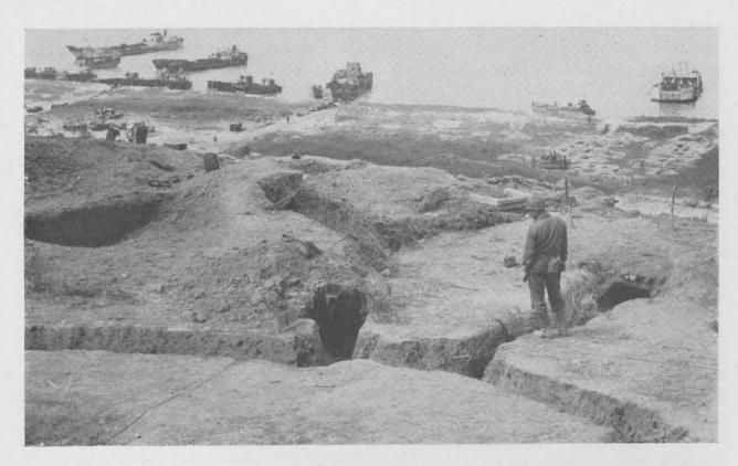
TRENCHES ALONG THE BLUFF EDGE were the main German defenses between strongpoints guarding draws. These trenches, leading from dugouts to firing positions, overlooked Easy Red Beach west of E-1 draw. Such systems usually included machine-gun positions.
