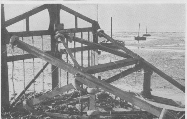
UNDERWATER OBSTACLES: Upper left, a mined post; upper right, hedgehog; below, Element "C" (with explosives attached for demolition by U. S. engineers who cleared the beaches). A fourth type found on Omaha, the log ramp, is seen in other illustrations.
